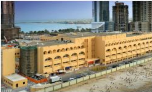
Corniche Maternity Hospital, Abu Dhabi, UAE
