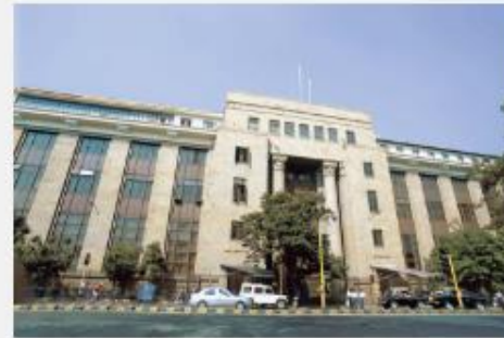
RBI Office Building (Old), Mumbai
