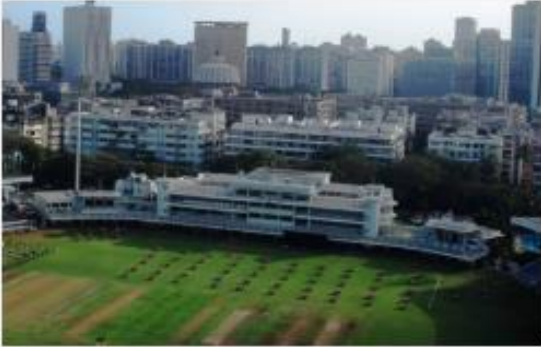
Brabourne Cricket Stadium, Mumbai
