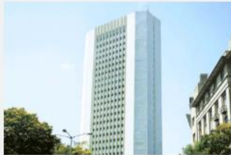
RBI Office Building (New), Mumbai
