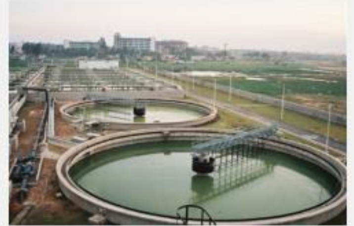
Sewage Treatment Plant, Kadabesinahalli, Bengaluru
