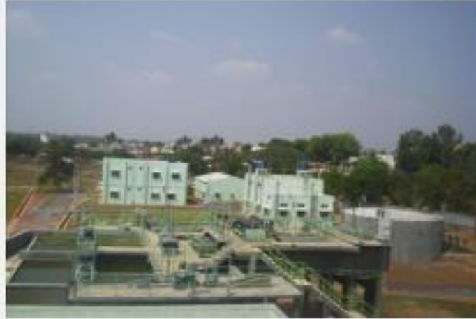
Sewage Treatment Plant, Nagasandra, Bengaluru
