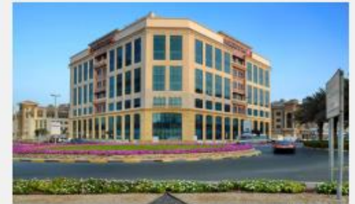
Sulaiman Al Habib Hospital, Dubai, UAE
